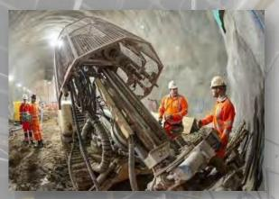
We offer a fleet of articulated mast drilling rigs which enable us to achieve full radial tunnel access for probe, ejector, TAMS and wellpoint drilling services. This coupled with bespoke in-tunnel pumping equipment has enabled us to deliver cost effective and efficient solutions for our customers
